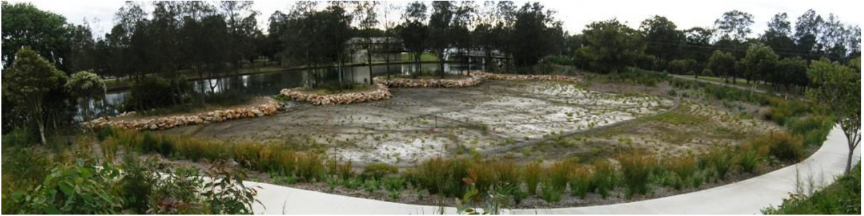
Saltmarsh Translocation in progress – Port Botany.
